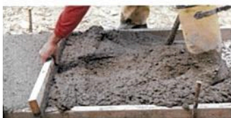
Hand Tools & Formwork
